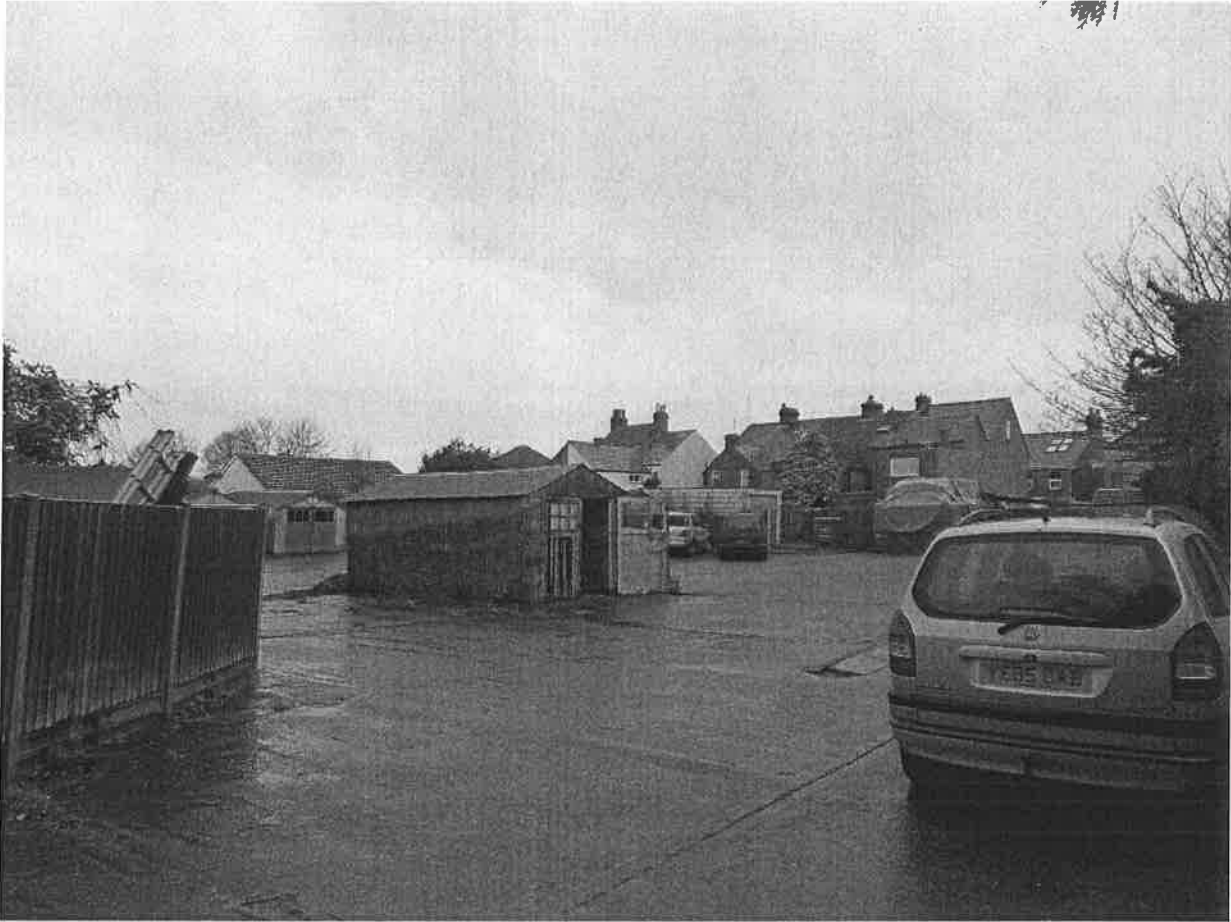
F/TH/14/0103 – Garages R/O 5 and 7 St Marys Road, Minster
